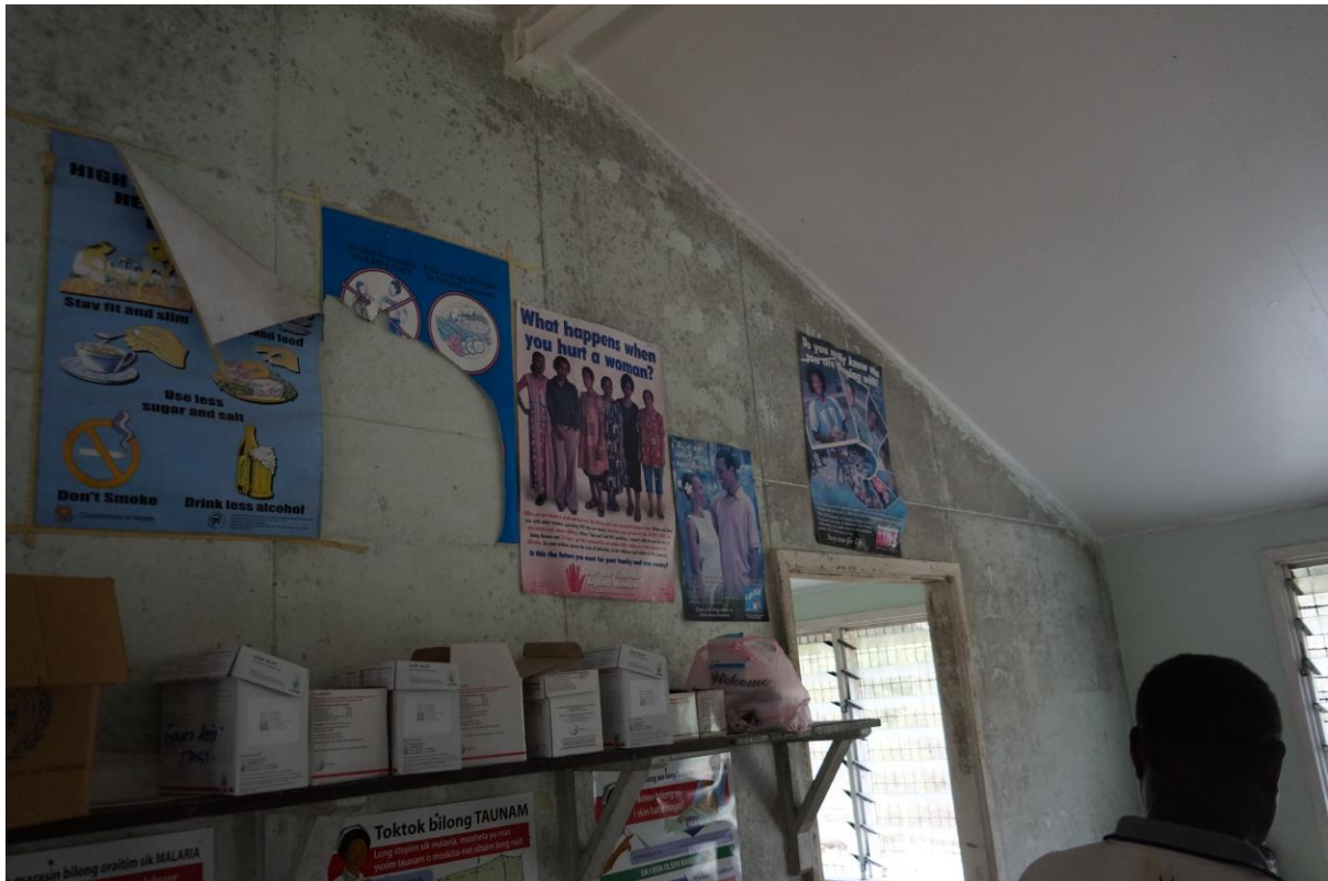
i The hospital was in poor condition before refurbishment, with rusted roofing iron, decaying floorboards and mouldy walls
