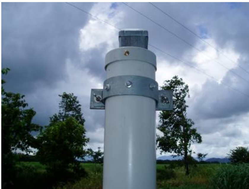
Figure 14 Close up of RSS clamp configuration.
