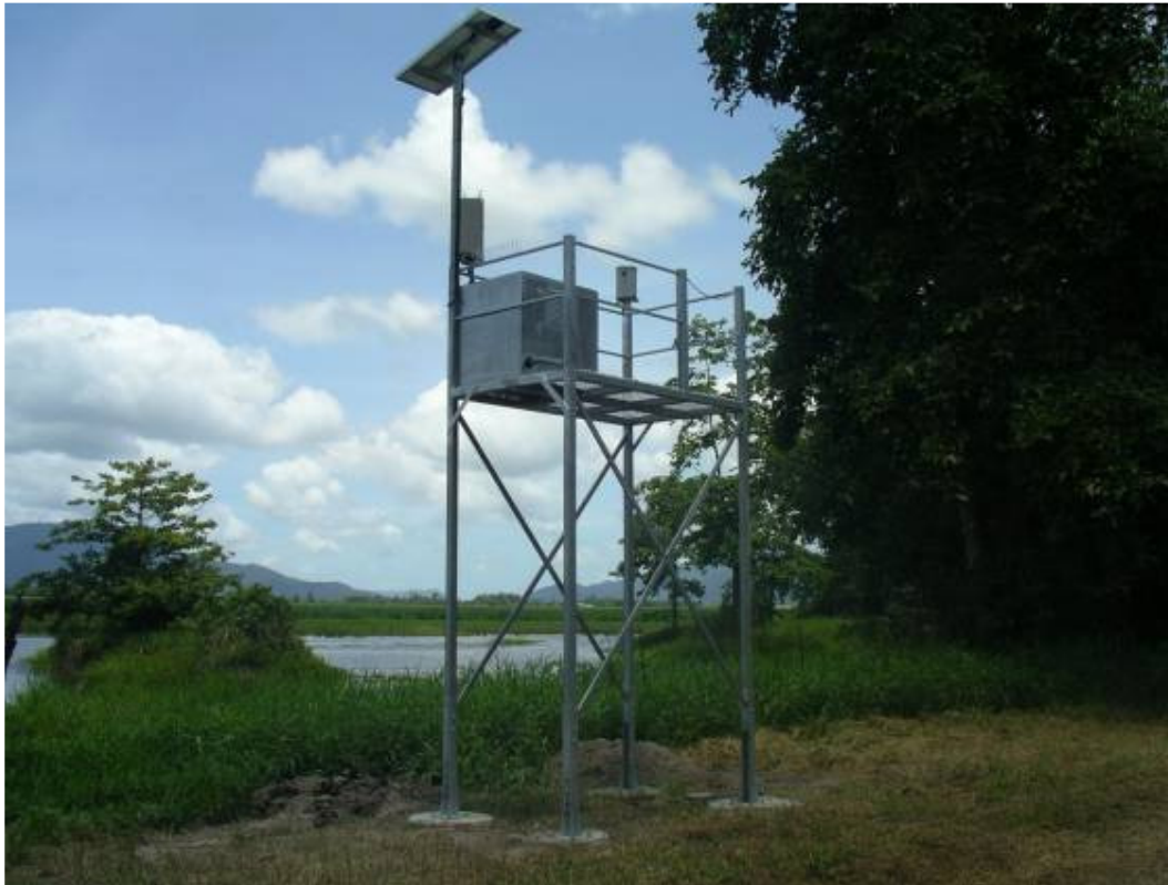
Figure 3 Fully automated flood monitoring station (S1) installed near the Murray River, Tully.
