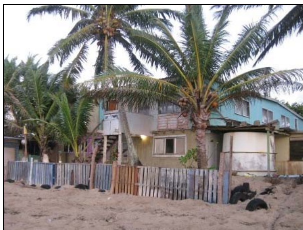
Figure 2: The use of crates, tyres and sandbags to protect a beachfront property on Erub Island. Photo by Karen McNamara.
