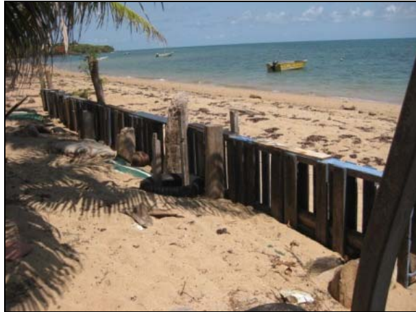
Figure 3: View of the crates, tyres and sandbags used to protect property. Photo by Karen McNamara.
