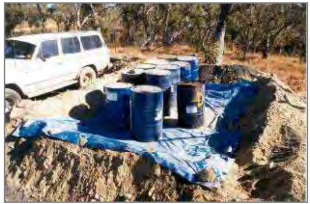
Temporary bunding can help to minimise the impact of road works (Photo: Guy Chester).
