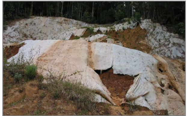
Poor maintenance of geofabric can result in erosion problems, weed invasions and failure of revegetation (Photo: Bruce Jennison).
