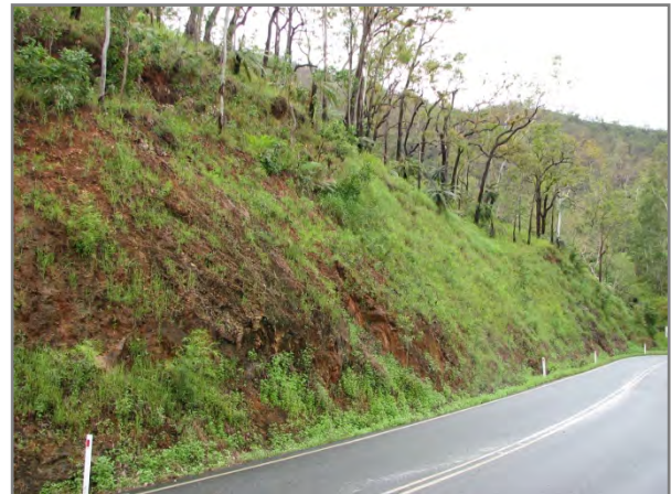
Hydromulching results at the same cutting on Gillies Highway ~ January 2006 (Photo: Nigel Tucker).
