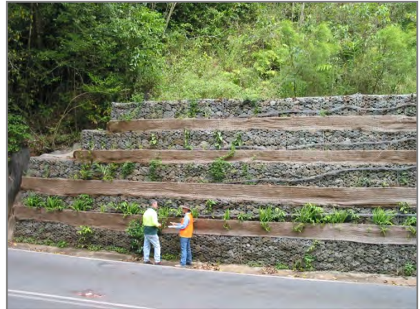
Rock-filled gabions act to retain cuts and fills, allowing steeper slopes, and hence less width of corridor disturbance (Photo: WTMA).
