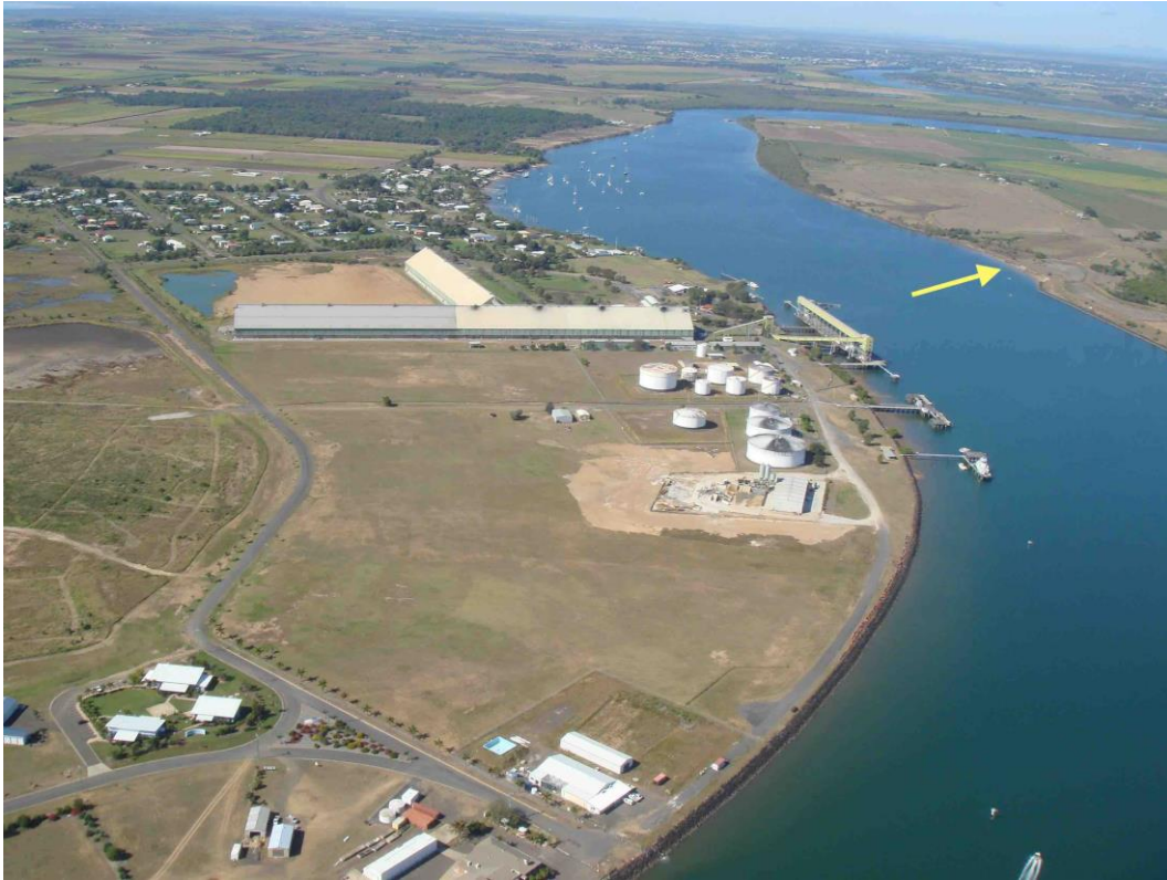
Figure 29: Burnett estuarine bank identified as in need of rehabilitation from the NESP Southern GBR project. The yellow arrow marks the location.
