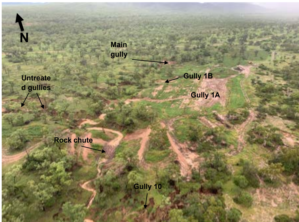
Figure 55: Image taken during sample collection for the January/February rainfall event (Photo credit: Damon Telfer). Note the area under the gully 1A text with little vegetation as a result of works to repair holes and tunnel erosion following the heavy rainfall in July (Source: NQ Dry Tropics)
