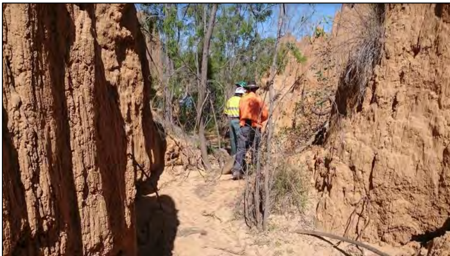
Slot canyon entrance of gully to channel, note undercut wall on left.
