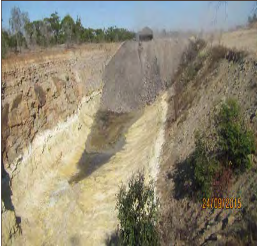
During - Garrick East Rehabilitation
