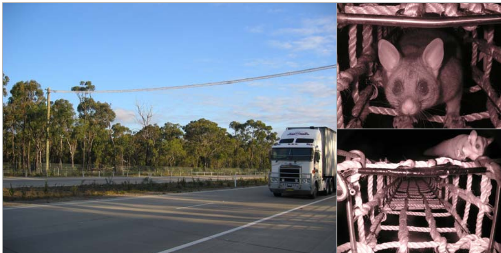
Figure 2.3 (Left) The long rope tunnel constructed by Thiess Pty Ltd over the divided four-lane highway at Karuah, near Newcastle, NSW, with (above right) brushtail possum and (below right) squirrel glider making use of it. Photos courtesy of Bob Bax.
