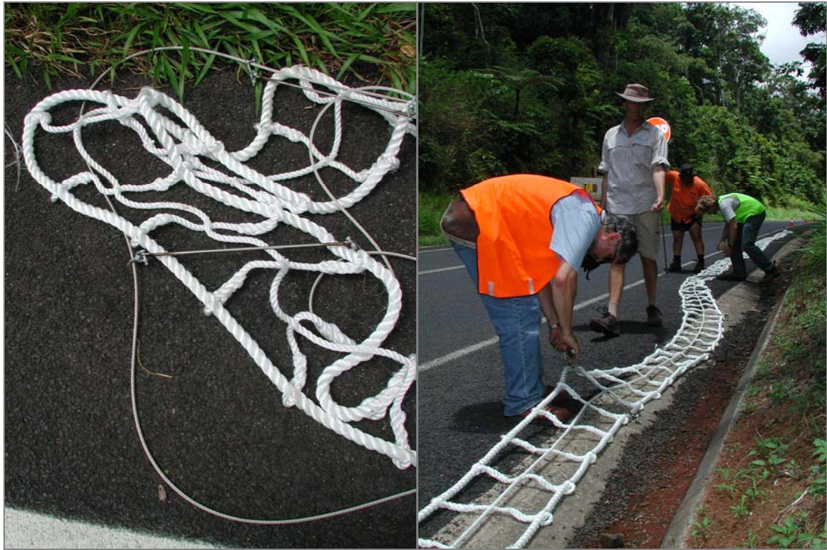
Figure 2.12 Rope ladder design showing finer rope cross-members spliced to 22 mm main length and stainless steel supports and attached to D-shackles threaded onto cable supports. Photos courtesy of Birgit Kuehn.
