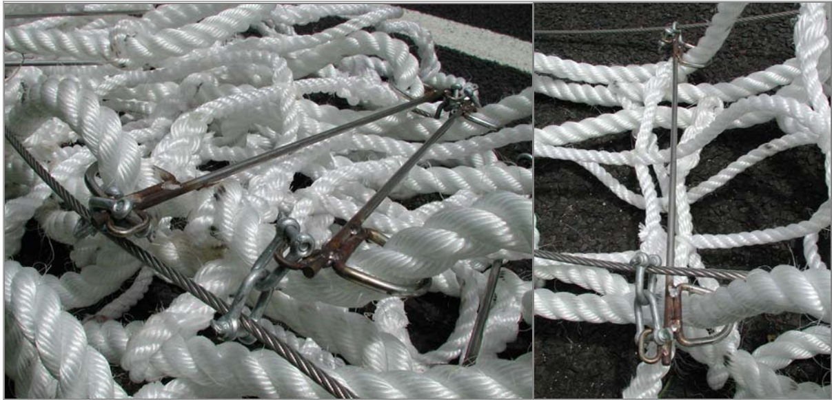
Figure 2.8 Rope tunnel showing ( left ) stainless steel framework and D-shackles attached to the cable, and ( right ) finer rope cross-members. Photos courtesy of Nigel Weston.
