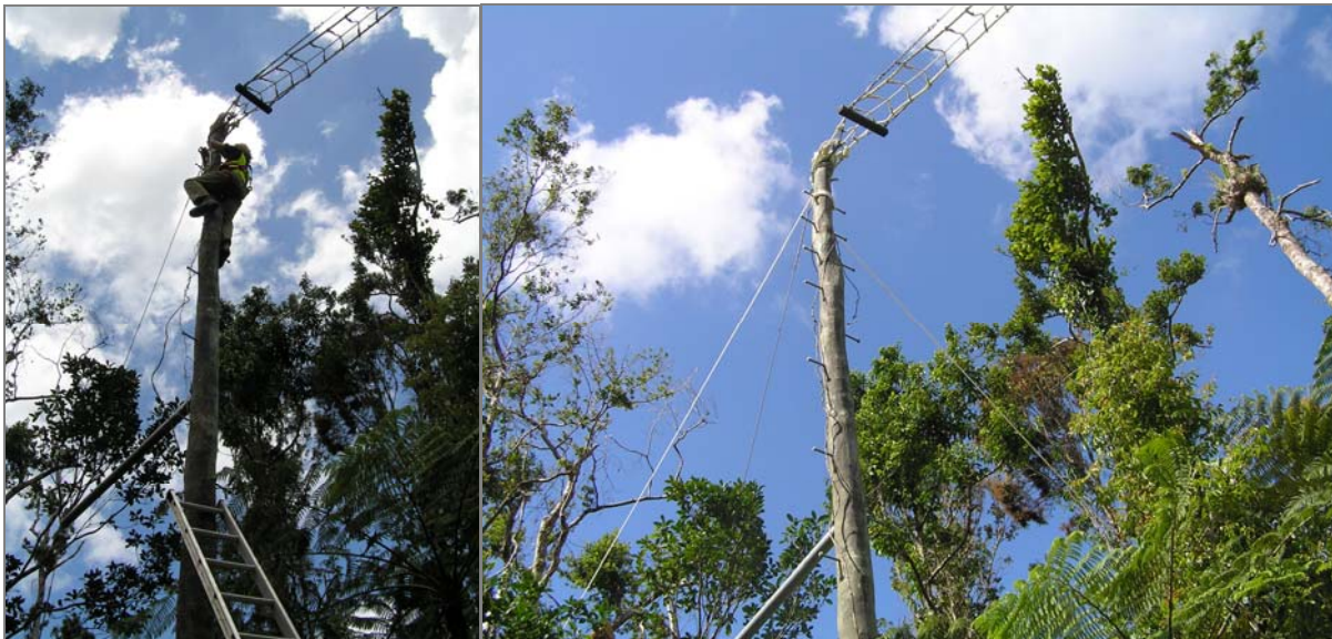
Figure 2.17 Installation of ropes from poles to neighboring trees, where poles were somewhat isolated from adjacent foliage. Photos courtesy of Miriam Goosem.
