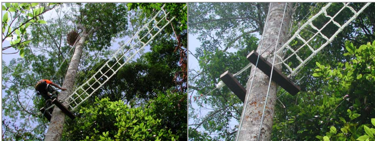
Figure 2.5 Canopy bridges were attached to trees using wooden supports to prevent damage to the tree. Photos courtesy of Birgit Kuehn.
