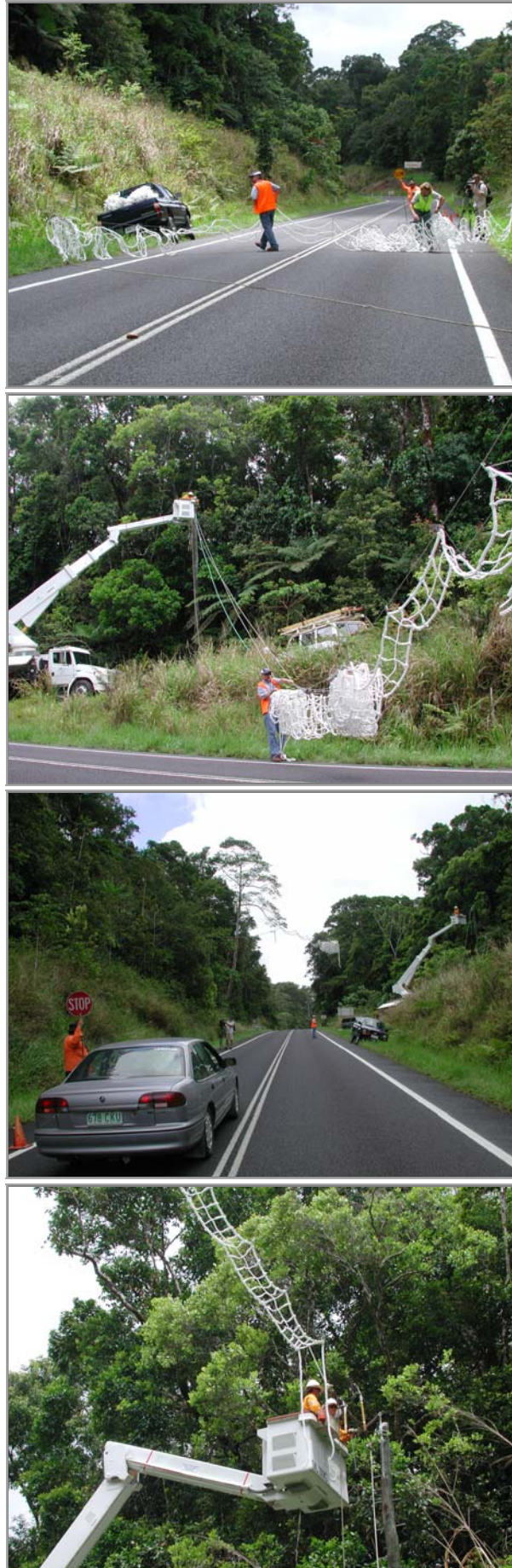
Figure 2.13 (cont'd) Erection of rope ladder canopy bridges. Photos courtesy of Birgit Kuehn.
