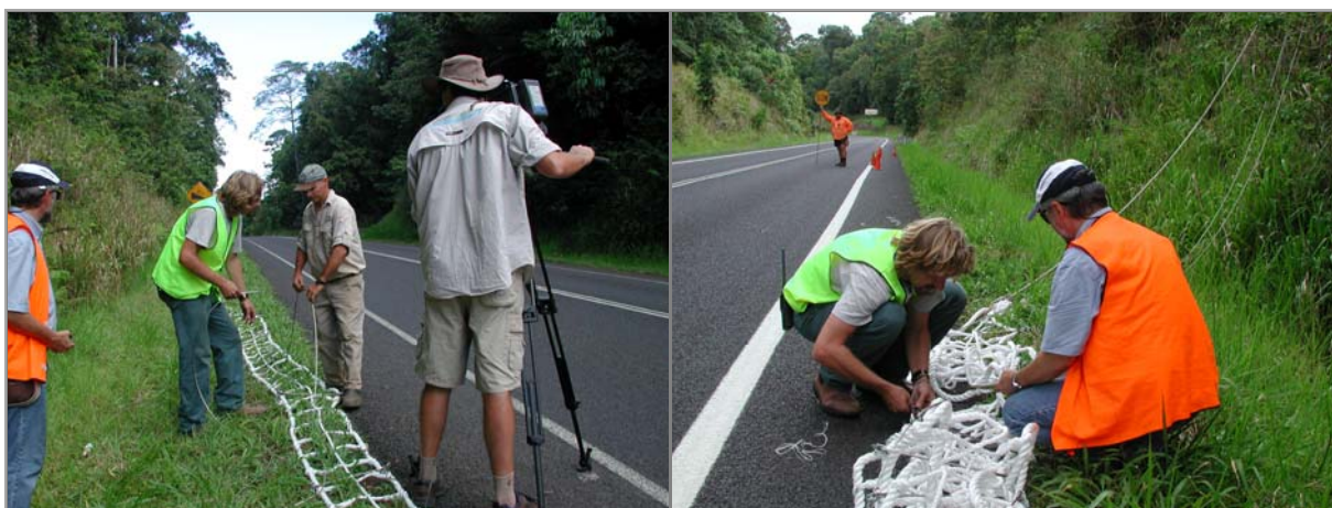
Figure 2.13 Erection of rope ladder canopy bridges. Photos courtesy of Birgit Kuehn.
