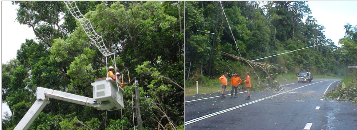
Figure 1.11 (Left) Attaching the rope ladder to telegraph pole, and (right) the rope ladder one month after installation after a tree collapsed on top of it. Photos courtesy of Robyn Wilson.
