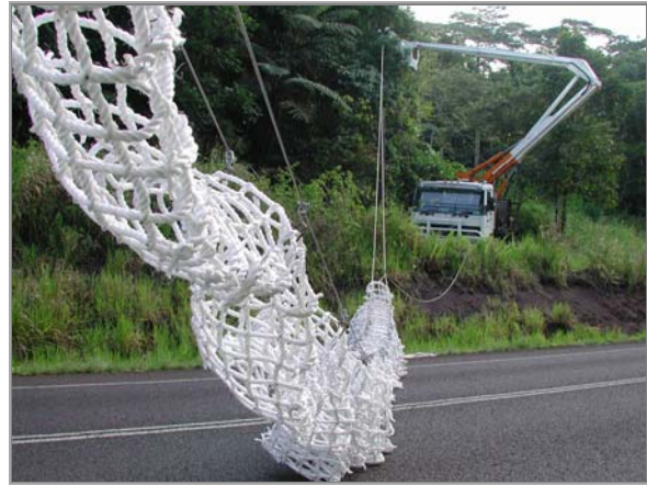
Figure 2.10 Ergon Energy cherry picker used to thread tunnel into position from electricity pole to tree support. Photos courtesy of Birgit Kuehn.
