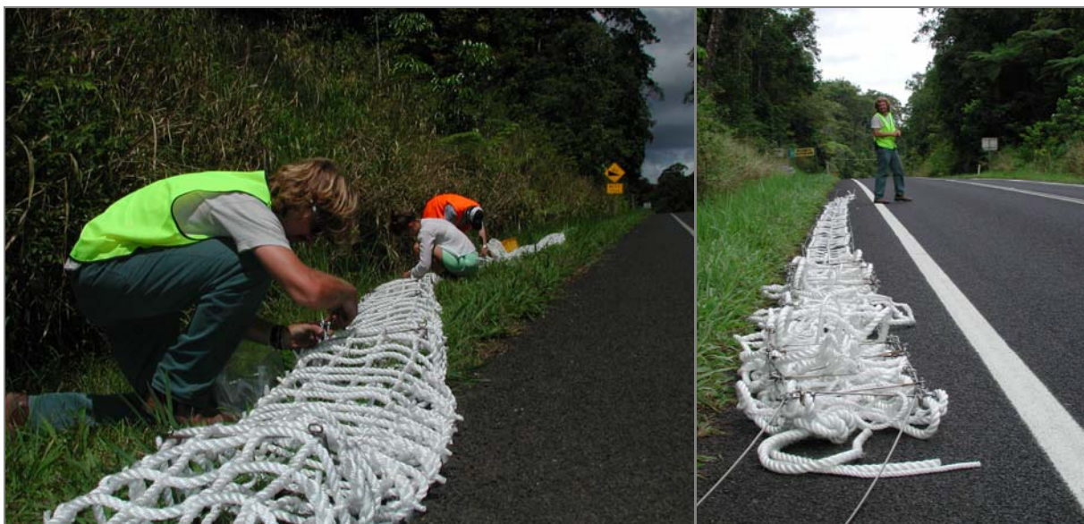
Figure 2.9 Attaching D-shackles and threading the cable for erection. Photos courtesy Birgit Kuehn.
