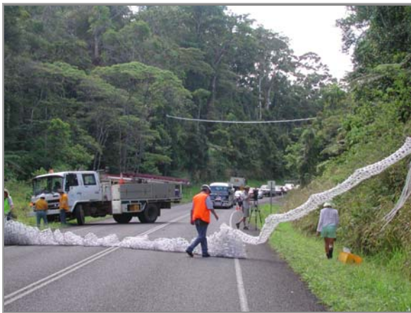
Figure 2.10 Ergon Energy cherry picker used to thread tunnel into position from electricity pole to tree support. Photos courtesy of Birgit Kuehn.
