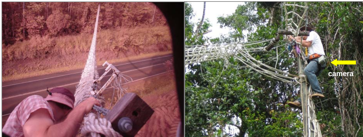
Figure 3.1 (Left) Installation of infrared-beam sensors on the rope tunnel canopy bridge, and (right) climbing the pole to the rope tunnel – note the camera housing ready to install, attached to the climber's hip. Photos courtesy of M. Cohen and J. Cooper.
