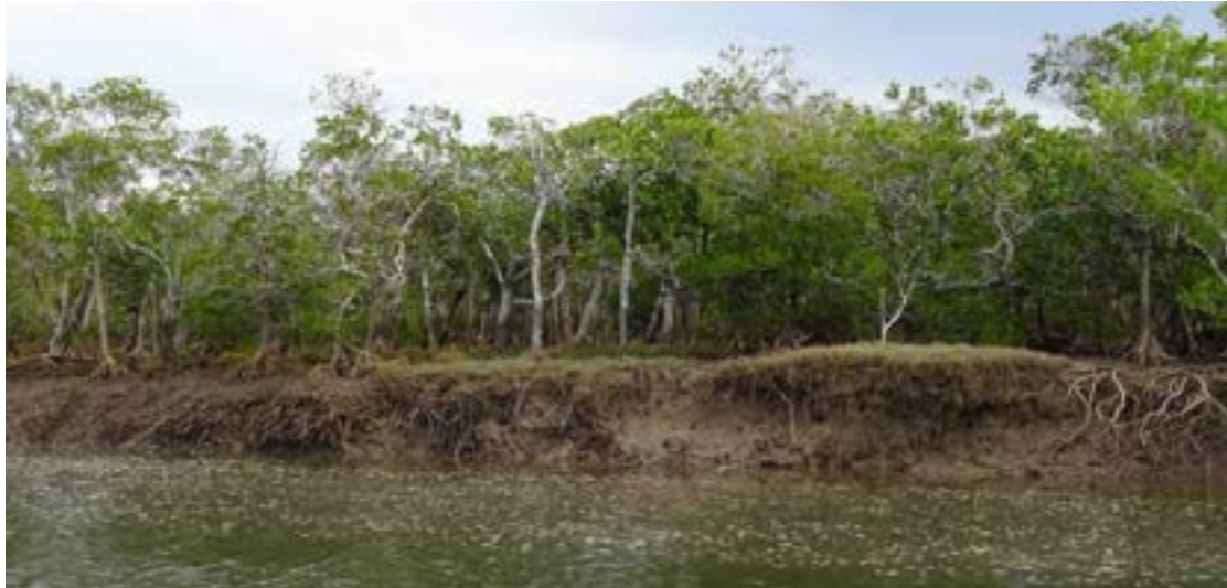
Figure 130: Bank erosion in the lower estuary with channel migration into upper-intertidal mangrove forest.
