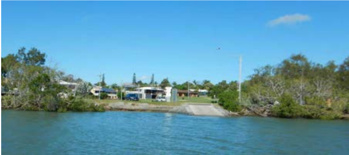
Figure 50: Boat ramps are common – so is the damage to connectivity and stability of estuary shorelines.
