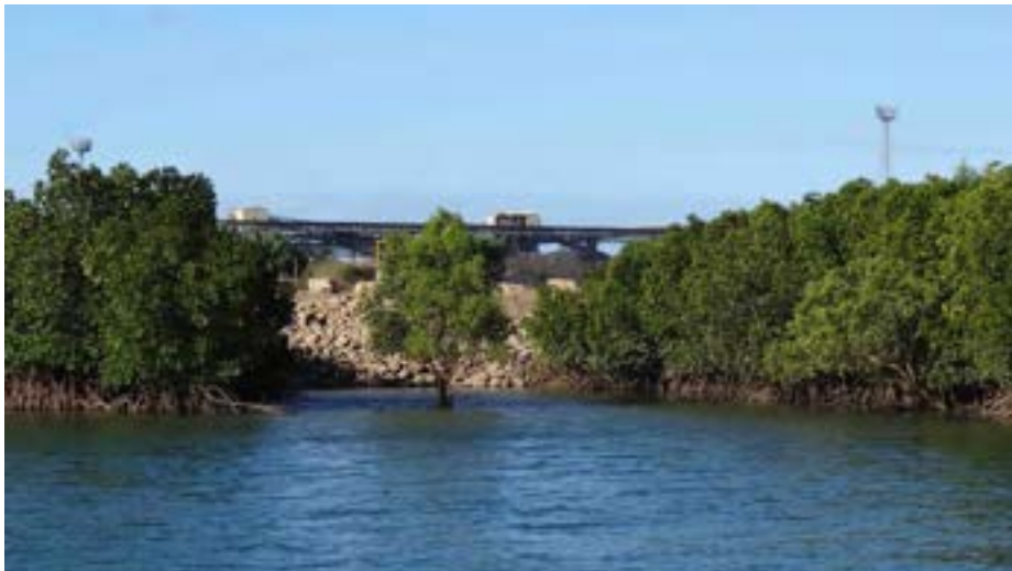
Figure 15: Landfill with bund wall blocks a natural drainage tributary altering the hydrology of the estuary.
