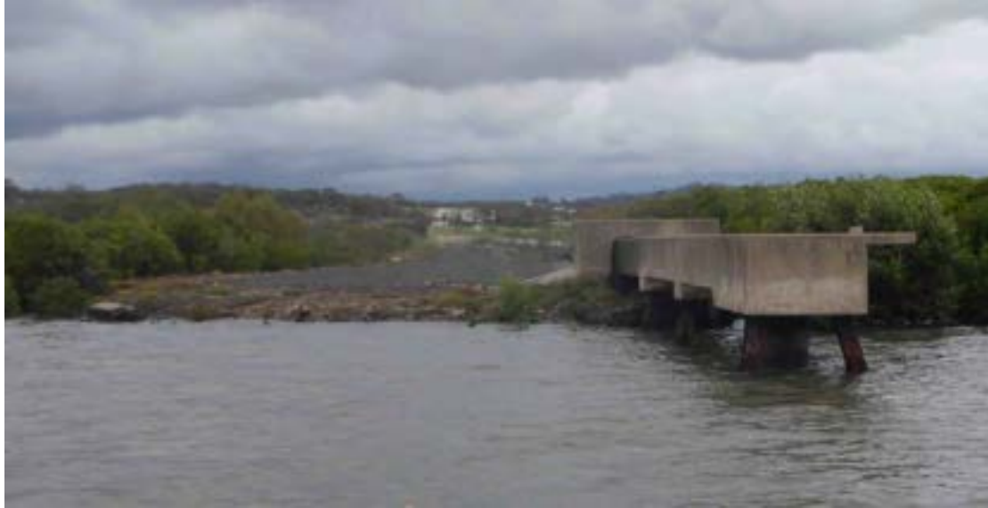
Figure 33: Damaged tidal wetland habitats are common adjacent to constructed structures needed for industry operations.
