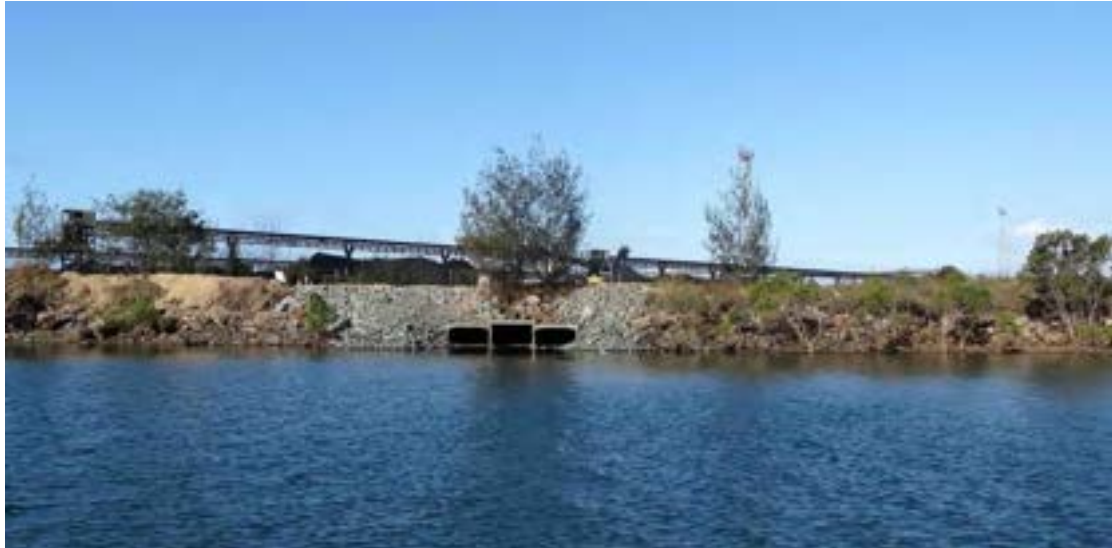
Figure 17: Drains along the landfill reclaimed areas are a feature downstream.
