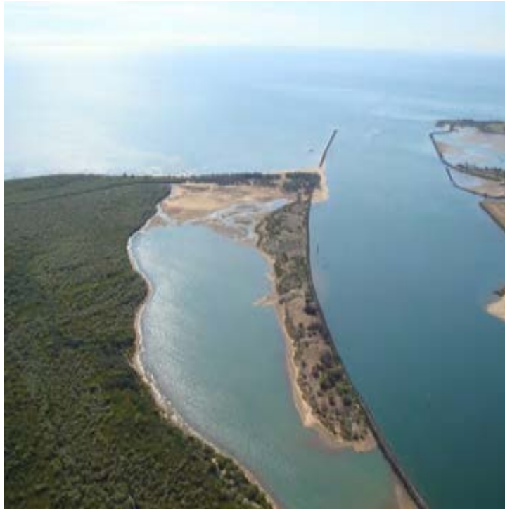
Figure 107: The training wall at the mouth of the Burnett River severely impacts natural flow.
