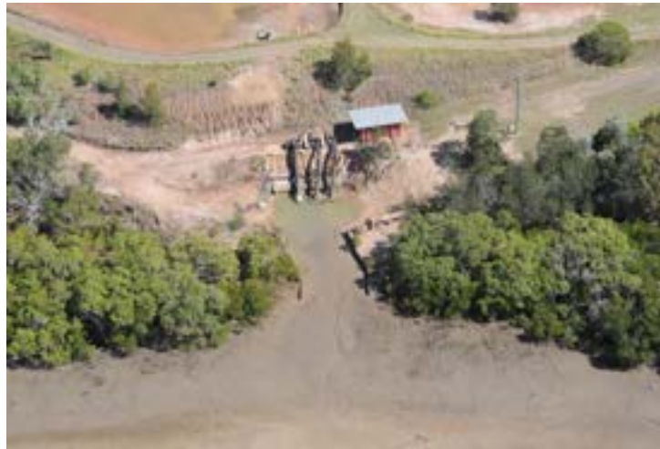
Figure 122: Mangrove removal for aquaculture intake/outlet pipes.
