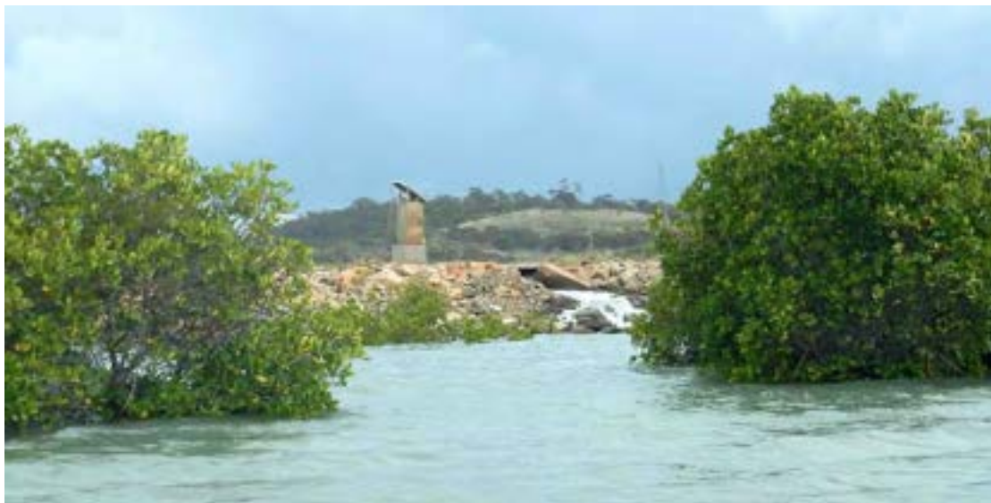
Figure 34: Constructed walls mark the perimeter of landfill areas with added drains from which flows unknown waste waters.
