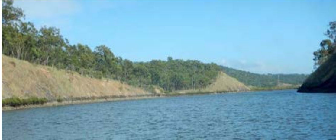
Figure 35: Channel modification has been undertaken on a massive scale in the channel connecting the inlet with Boyne estuaries.
