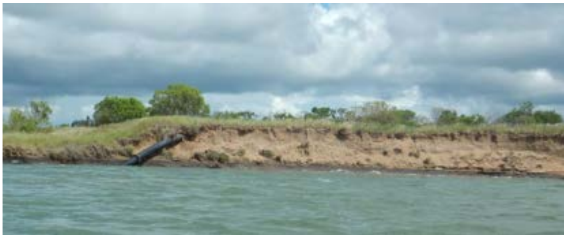
Figure 109: Bank erosion associated with wave action undermining unconsolidated shorelines downstream in the Burnett estuary.
