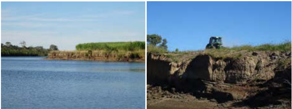
Figure 91: The absence of a riparian buffer and cropping to estuary margins increases erosion risk and estuary sediment loads.
