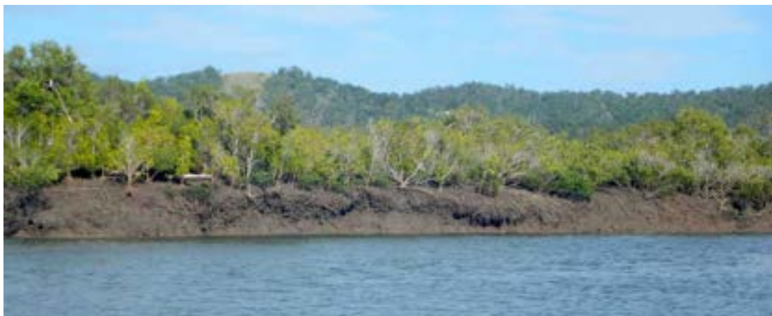
Figure 38: Bank erosion and slumping is not too common in the estuary.
