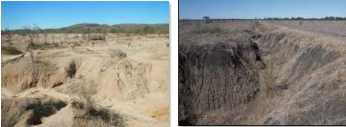
Figure 39: Examples of a gully in a Uniform Soil Material Group
