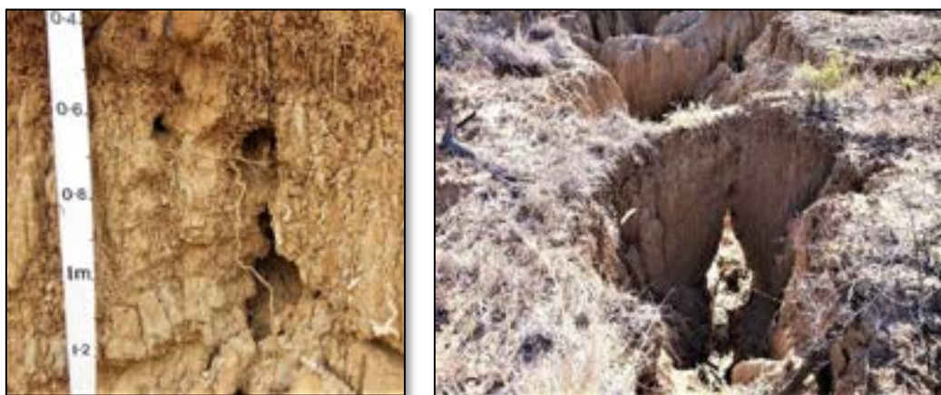
Figure 48: Examples of tunnel erosion in gully walls.
