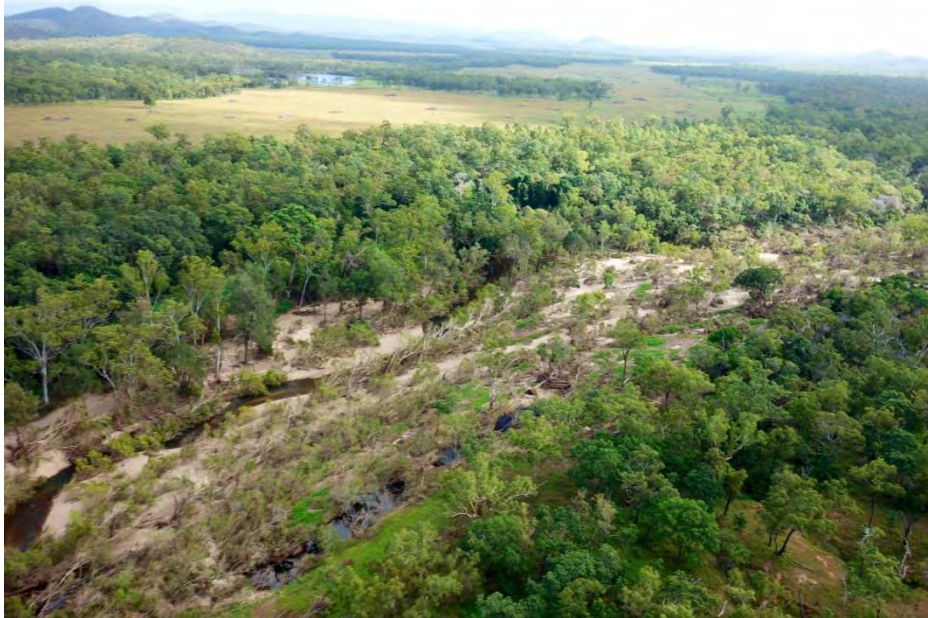
Figure A7: East Normanby River in the immediate aftermath of the flood generated by Cyclone Ita (photo Tim Hughes).
