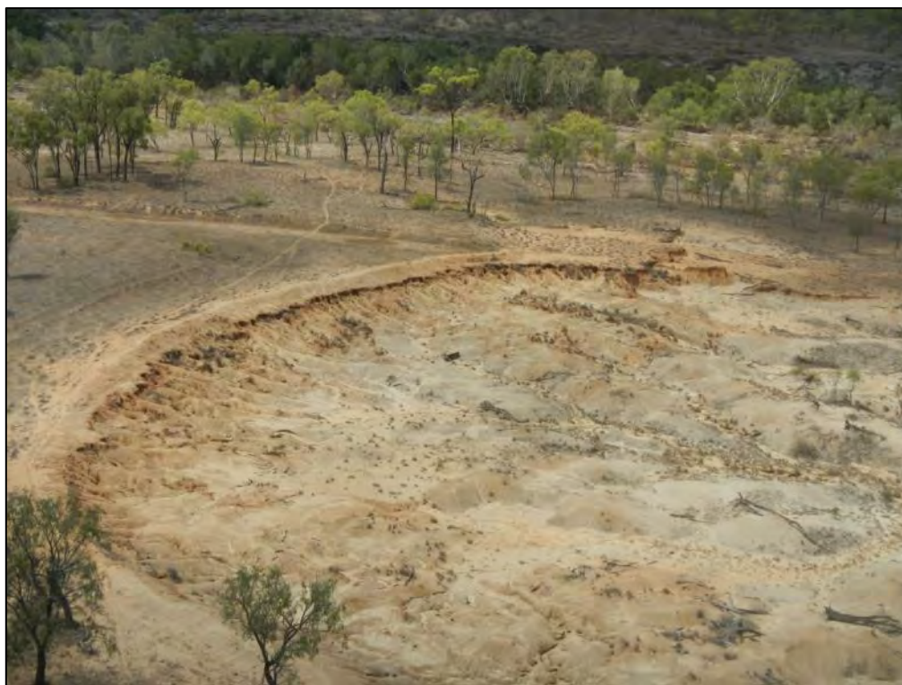
Figure 37: Example of a regraded alluvial gully in the Bowen catchment of unknown age with a constructed berm to exclude overland flow from the gully and with no soil treatment. This is the equivalent of the plot 1 control site - in which the gully is regraded with only direct rainfall driving high levels of ongoing erosion.
