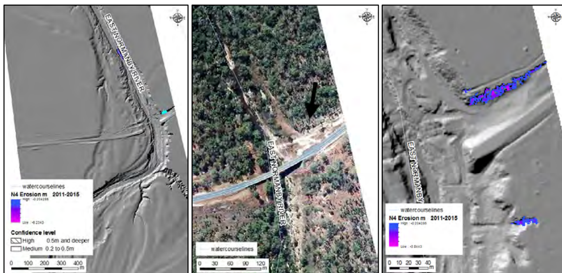
Figure A42: Fourth largest patch of erosion into ancient flood plain is associated with a road crossing the East Normanby, volume of erosion was 355m 3 in total.
