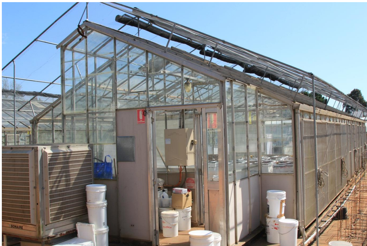
Figure 4. Glasshouse in Toowoomba
