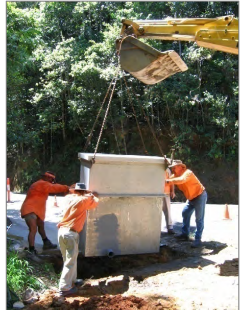
Installation of runoff water treatment system on rainforest highway, northeast Queensland (Photo: Bernd Lottermoser).
