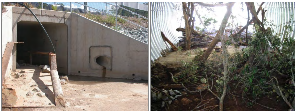
( Left ) Faunal underpass constructed at Compton Road, Brisbane, targeted at wallabies, possums, koalas, reptiles and amphibians. Note, the ledges about one metre high for small mammals and logs erected at the same height for koalas and possums. The ledge allows dry passage for animals away from the water carried by the culvert (Photo: Brisbane City Council). ( Right ) Interior of faunal underpass near Millaa Millaa, northern Queensland, with rocks, logs and brush for cover from predators for ground-dwelling animals, and vertical poles erected for escape from predators for tree-dwelling animals (Photo: Miriam Goosem).
