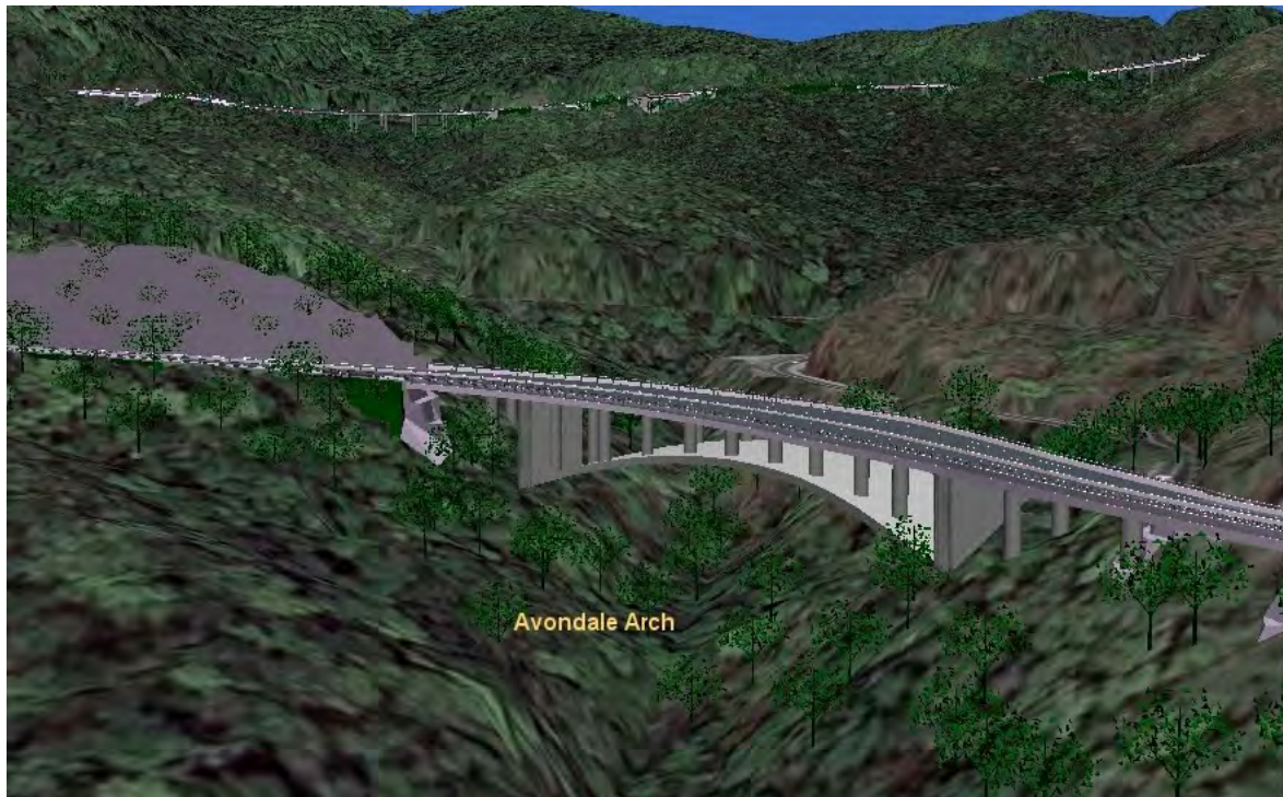
An artist's diagram of a high bridge over the rainforest canopy proposed for the Kuranda Range Road upgrade project. Note, tree canopies below the arch (Diagram: Queensland Department of Main Roads 2005).
