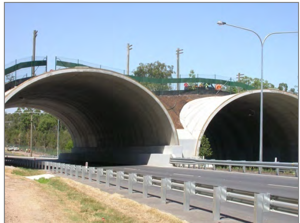
( Left ) Low bridges can provide dry passage for ground-dwelling animals during most of the year. Maintaining vegetation under the bridge, together with rocks and logs, will promote animal use of the area (Photo: Miriam Goosem). ( Right ) Land bridge built at Compton Road, Brisbane. Note, depth of soil for vegetation plantings, fencing to prevent fauna jumping onto the road surface, glider poles for movements of glider possums and escape from predators by arboreal species (Photo: Brisbane City Council).
