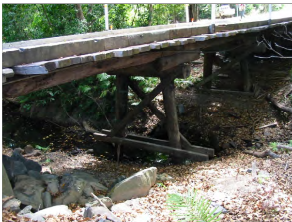
( Left ) Low bridges can provide dry passage for ground-dwelling animals during most of the year. Maintaining vegetation under the bridge, together with rocks and logs, will promote animal use of the area (Photo: Miriam Goosem). ( Right ) Land bridge built at Compton Road, Brisbane. Note, depth of soil for vegetation plantings, fencing to prevent fauna jumping onto the road surface, glider poles for movements of glider possums and escape from predators by arboreal species (Photo: Brisbane City Council).
