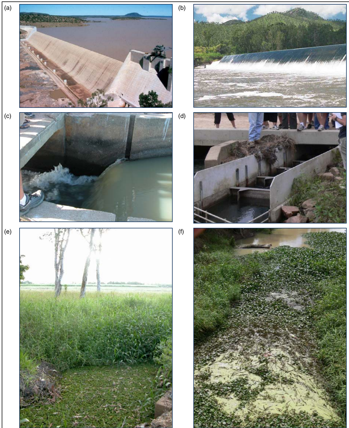
Figure 4: Connectivity issues: (a) dams (Burdekin Falls); (b) weirs (Ross River); (c) drop boards (d) fish way around drop boards; (e-f) blockage of waterways by invasive plants; (c-f) located on the Burdekin floodplain. Photographs courtesy of R. G. Pearson.
